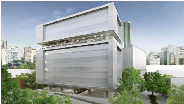
Fig 1. Perspective of the new building under construction which includes a clean room class 1000.
