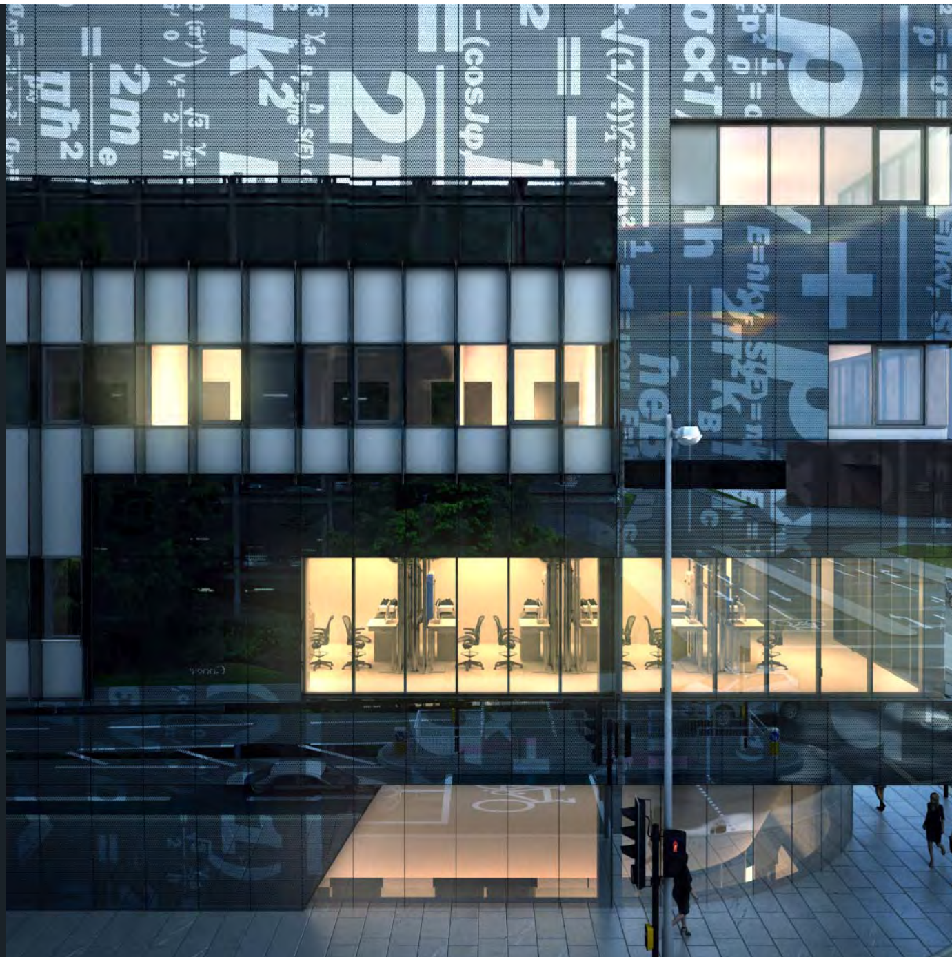
East Façade Detail
