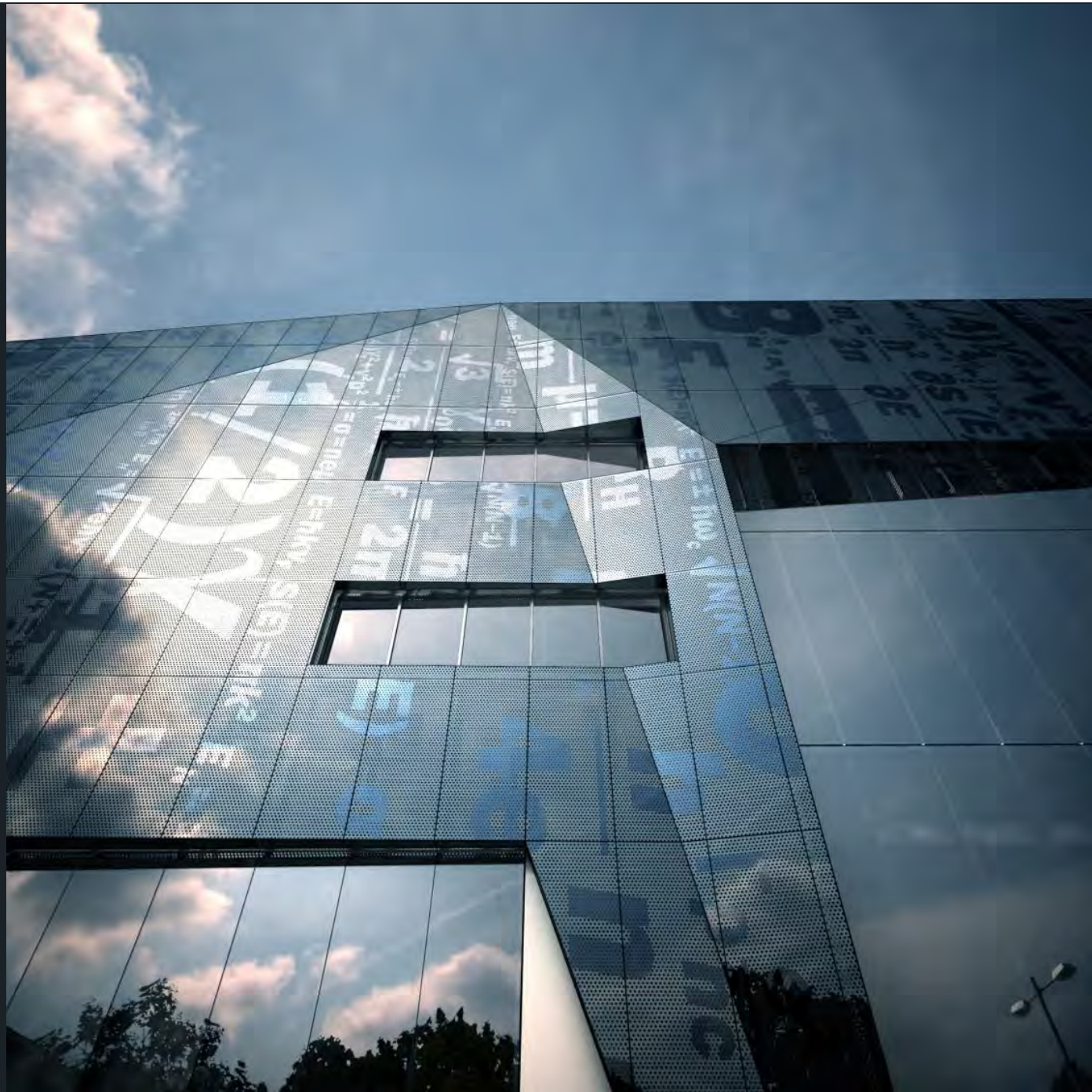
North Façade Detail
